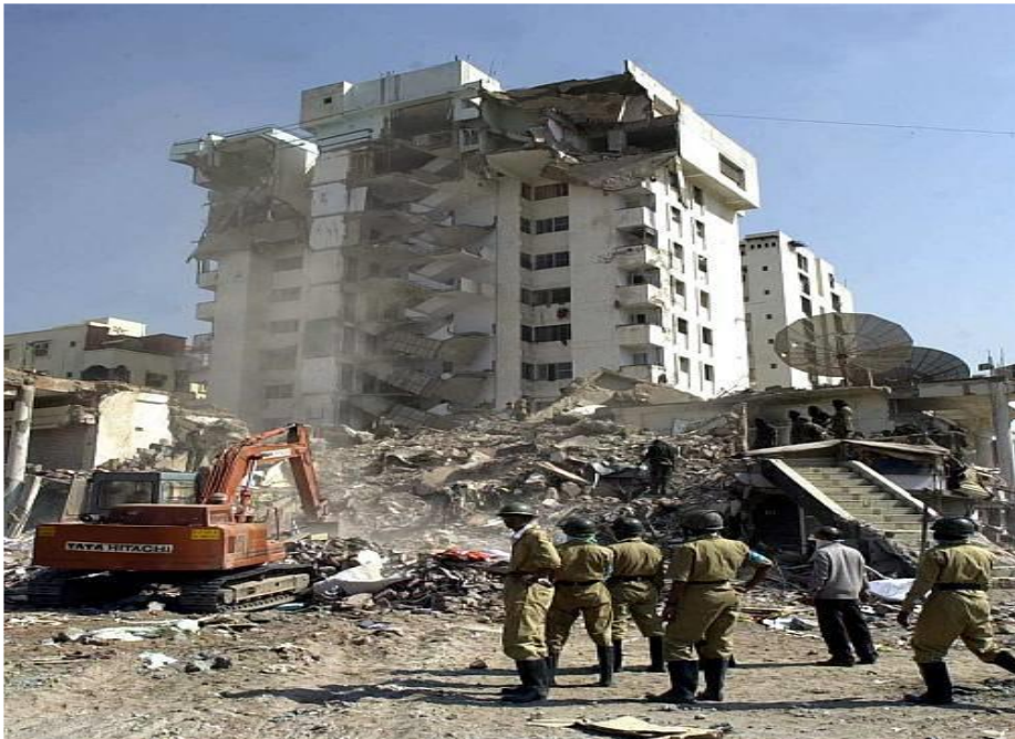
Figure. 2: Apartment collapse in Bhuj
