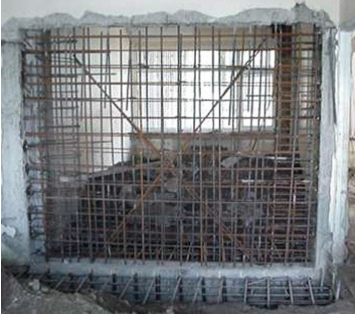
Fig 2: Additional Shear Wall
