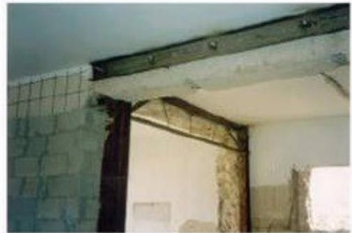
Strengthening by steel plates.
