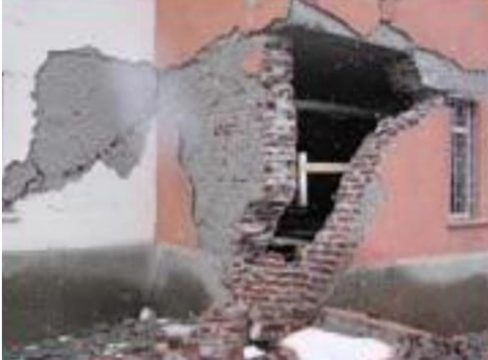
Fig: Corner Failure of Masonry Wall
