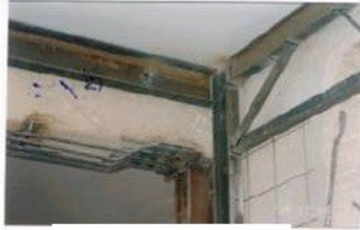
Strengthening a beam and Slab.
