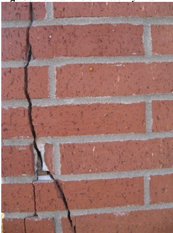
Fig: Corner Failure of Masonry Wall
