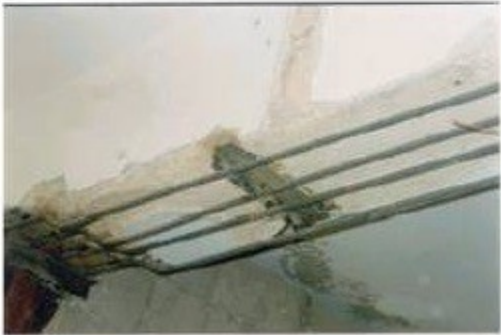
Jacketing a beam by increasing bars and cross section.
