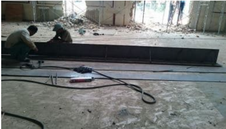
Fig. 4: Welding steel jacket
