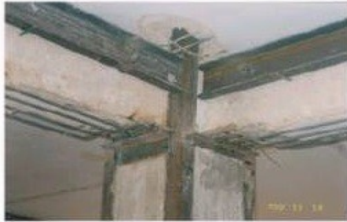
Strengthening a beam , slab and column.
